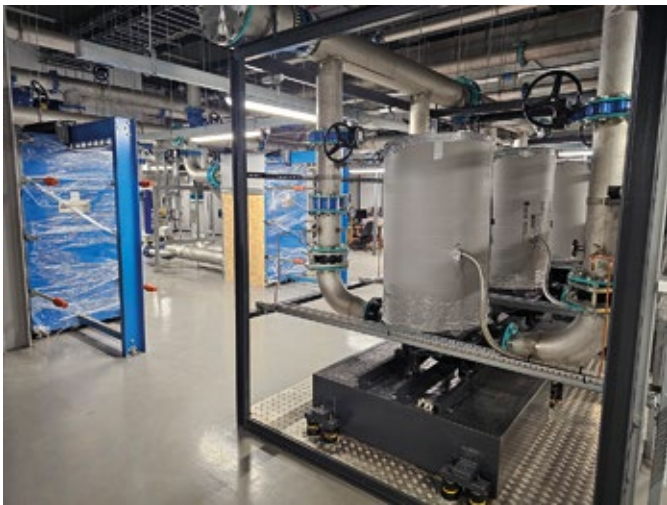
These photographs show spaces at the ACF which are being prepared for the arrival of the Next National Supercomputing Service.
